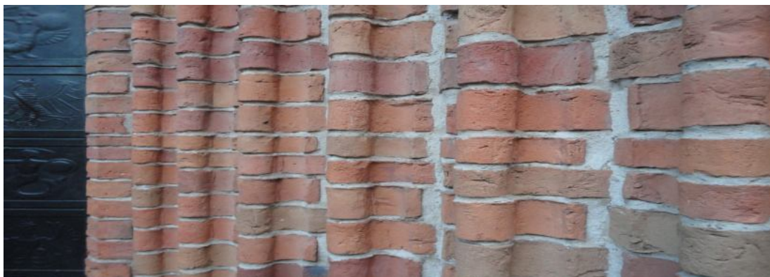
The munkensten brickwork typology.
